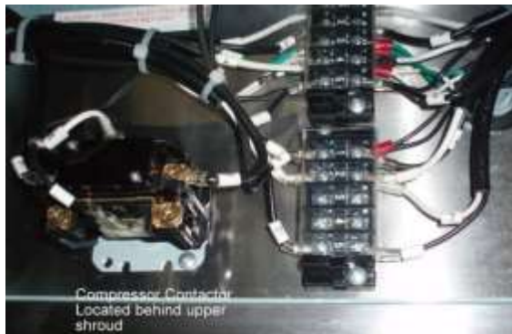
Compressor Contactor
